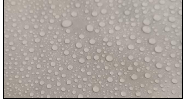
Figure 2: CIKOMicro Topping sealed with water repellent
